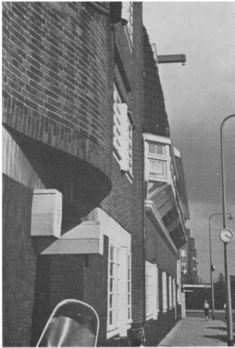
Fig. 31 THIRD BLOCK: EXTERIOR DETAIL ALONG ZAAANSTRAAT. Photograph: Dick Frank, New York.
