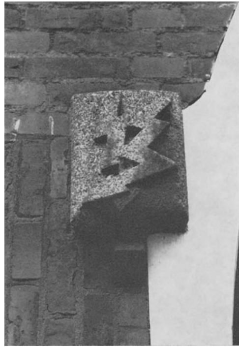
Fig. 38 THIRD BLOCK: EXTERIOR DETAIL; ORNAMENT AT IMPOST OF WINDOW OF POST OFFICE ON OOSTZAANSTRAAT. Photograph: Dick Frank, New York.
