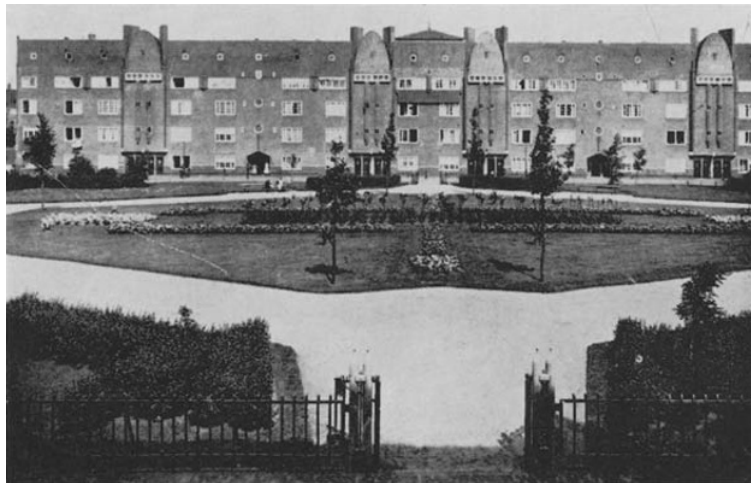
Fig. 6 FIRST BLOCK; PLANTSOEN FAÇADE WITH VIEW OF PARK IN FOREGROUND, ca. 1920. Photograph: 'Stichting Lichtbeelden-Instituut' Amsterdam.
