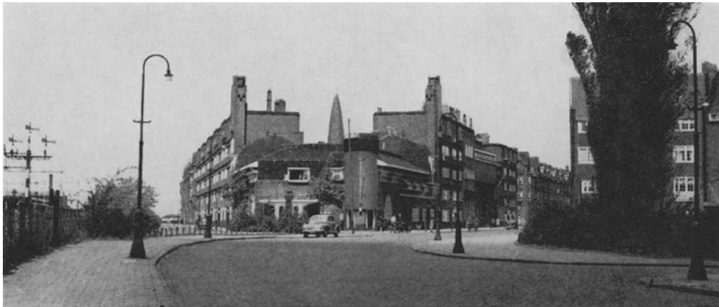
Fig. 3 SPAARNDAMMERBUURT; THIRD BLOCK ALONG ZAAANSTRAAT, AT APEX OF TRIANGULAR SITE LOOKING NORTH. April, 1958.
