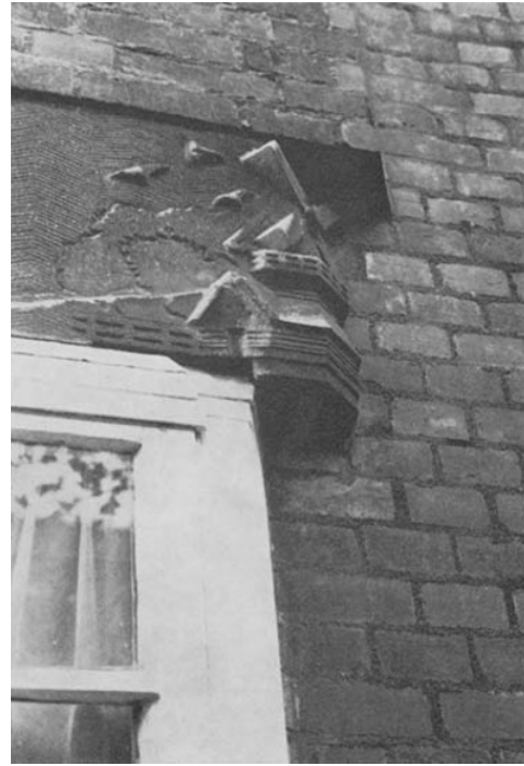
Fig. 36 THIRD BLOCK: EXTERIOR DETAIL; WINDMILL ORNAMENT ON ZAAANSTRAAT. Photograph: Dick Frank, New York.
